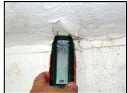
3.2 Picture 3 No heightened level of moisture in that area
