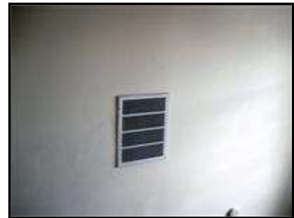
8.1 Picture 6 Return air vent high on wall above stairs. Not inspected.
