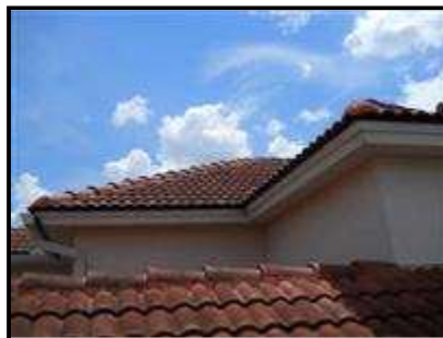
1.1 Picture 11 North side, looking South
