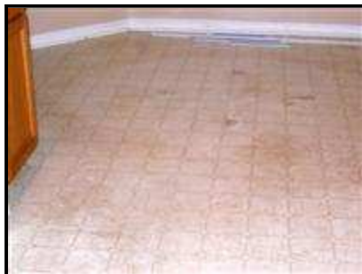
4.3 Picture 14 Same here.
