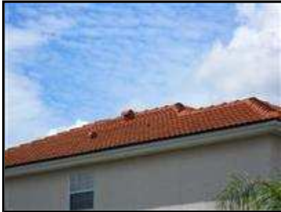
1.1 Picture 16 South side, looking NW.
