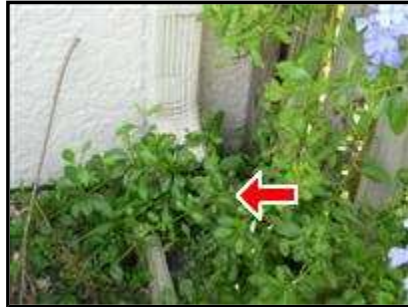
1.2 Picture 7 Splashblock needed here
