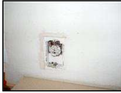
7.0 Picture 2 Replace cover for this low voltage component.
