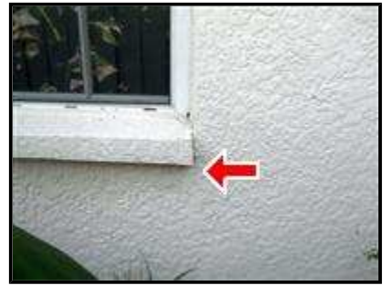
2.1 Picture 13 North side window at garage.
