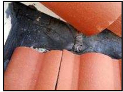
1.1 Picture 3 Field tiles below previous picture tiles which are sliding down toward the gutter thus revealing underlying flashing and tar.
