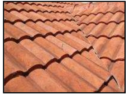
1.1 Picture 15 Valley over garage.
