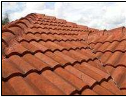
1.1 Picture 13 East side over garage.
