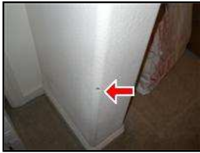
4.2 Picture 10 Master closet area
