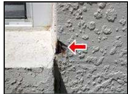
2.1 Picture 7 Patch & paint - same window
