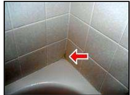
4.2 Picture 3 Upstairs guest bath - repair caulk/grout lines
