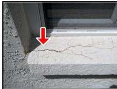
2.1 Picture 6 Repair sill at previous picture
