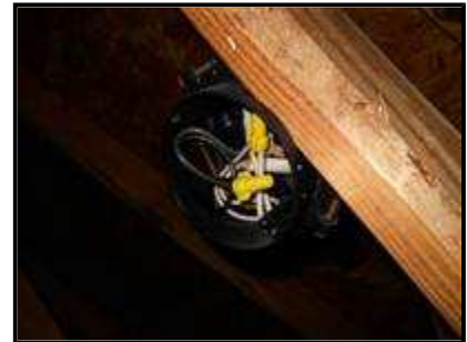
7.4 Picture 3 Attic over garage
