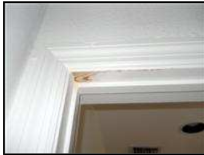
4.6 Picture 1 SE corner, upstairs bedroom
