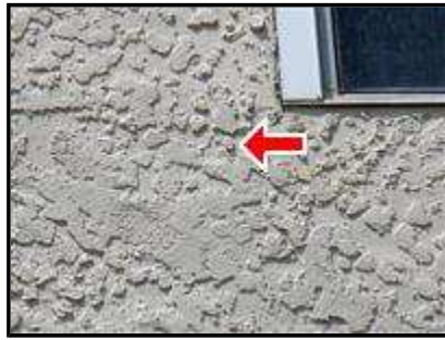
2.1 Picture 1 South side, upper story
