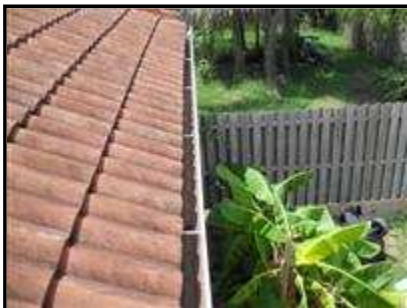
1.2 Picture 1 Gutters are clear
