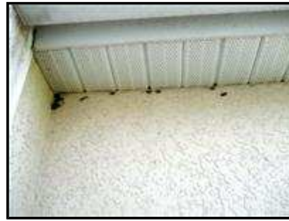
2.9 Picture 5 Right of front entry.
